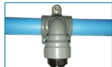
Step 6: Fixing the Droplet on the tube
